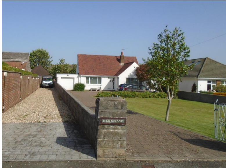
Figure 1 Photograph of the existing front elevation of the application building
